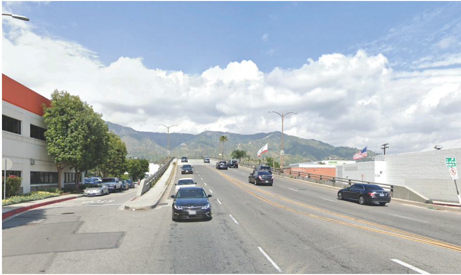
FIG 3.16 EXISTING PROJECT AREA 2 (VIADUCT) – LOOKING NORTH
