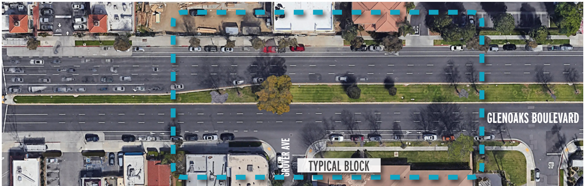
FIG 2.16 TYPICAL BLOCK EXISTING CONDITION (GLENOAKS BOULEVARD AND GROVER AVENUE)
