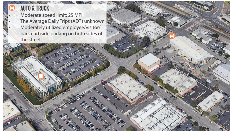
FIG 3.27 EXISTING PROJECT AREA 2 SAN FERNANDO ROAD TO FLOWER STREET – LOOKING NORTH
